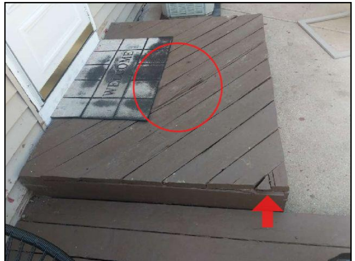
Soft boards/ damaged end piece
