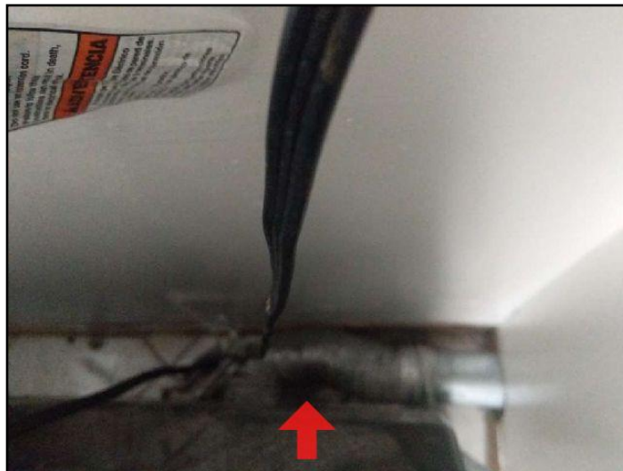
Dryer vent material not smooth wall
