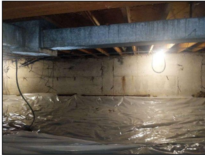
Uninsulated supply duct
