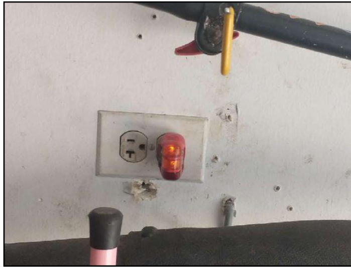
GFCI/GFI needed (Ground Fault Circuit...
