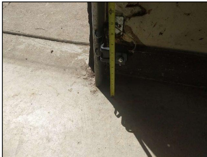
Sensors poorly located
