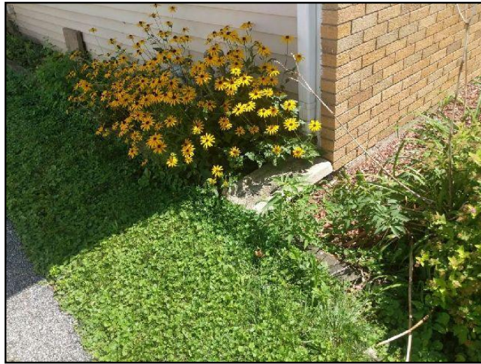
Should discharge 6 feet from building
