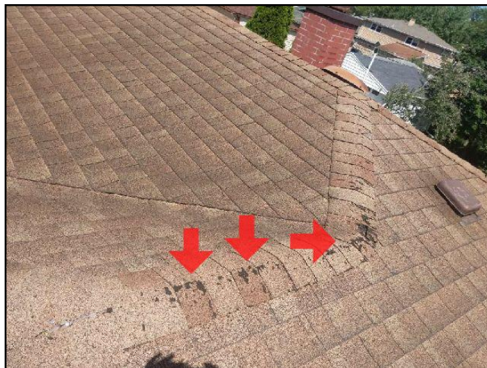
Ridge shingle deterioration
