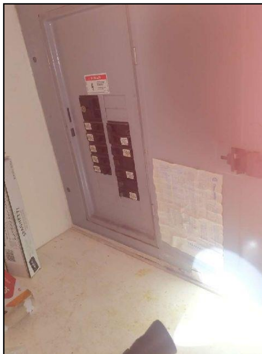
The circuits are not labeled at the panel
