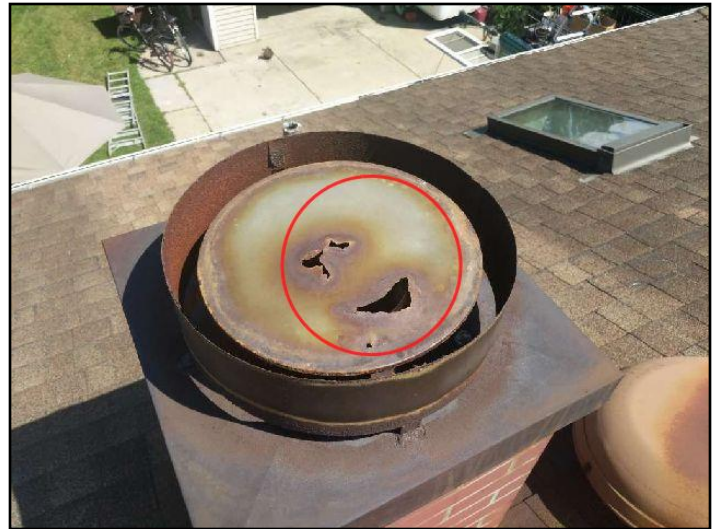
Hole in top of faux chimney
