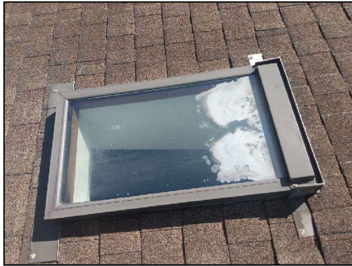
Thermo seal broken
